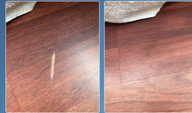
Engineered flooring was scraped on delivery, repaired with colour matching paint and detailed the grain to near original condition. Lacquered for finish, customer approved.
